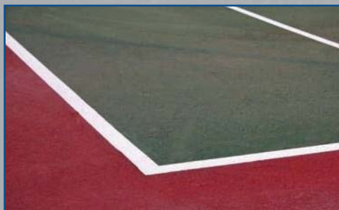
RiteWay Crack Repair System: Finished repair.
