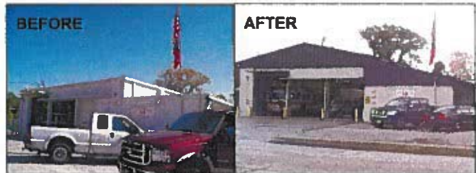
City of Houston Fire Station 38
