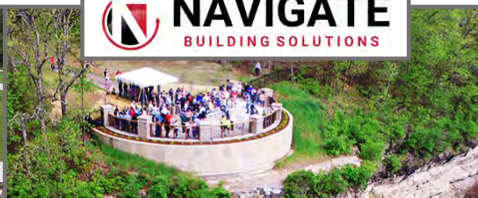
3-40 feet tall Retaining Walls
