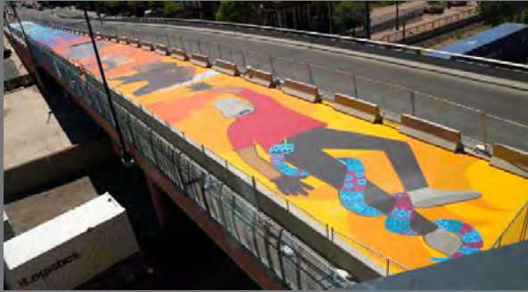
El Paso Chihuahuas - Pedestrian Bridge coating
