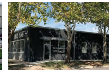
WICHITA, KS OFFICE
