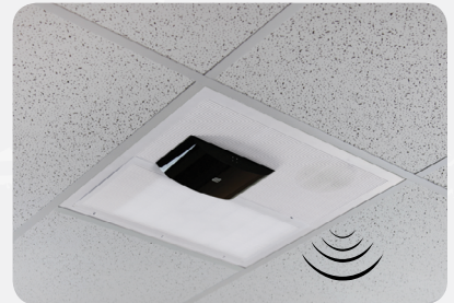
TOPCAT ceiling installation
