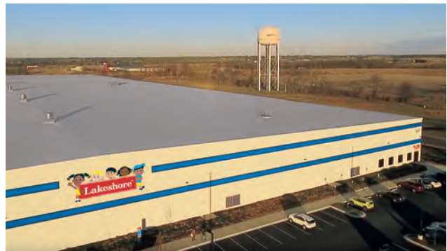
Our eastern distribution center in Midway, Kentucky.
