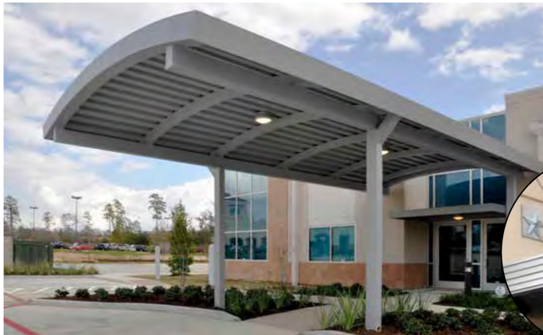
Creekside Surgery Center, Browne McGregor Architects
