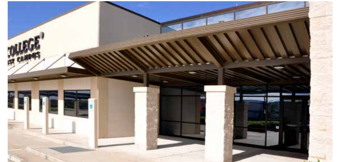
Remington College, Browne Penland McGregor Stephens Architects
