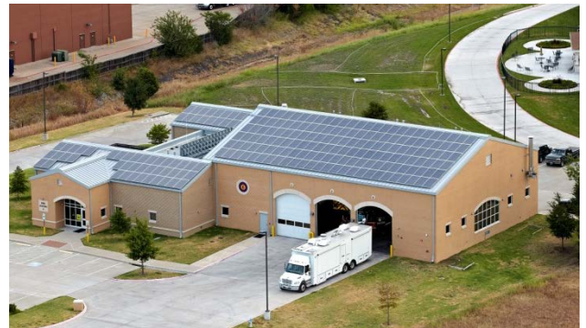
City of McKinney Fire Station – 52 kW
