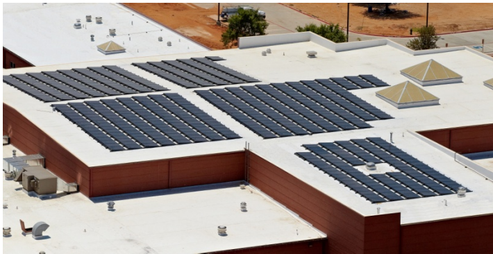
Bridgeport ISD High School – 170 kW
