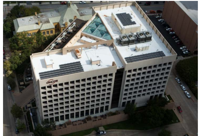
Oncor Electric Delivery – 42 kW
