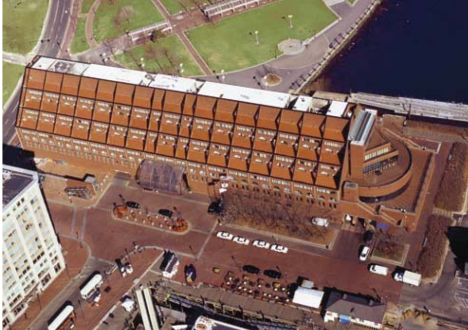
The re-roofing of a local Boston landmark in 2005, the Marriott Long Wharf hotel, presented Sika Sarnafil with the opportunity to conduct one of the first vinyl roof recycling projects in the U.S. The hotel's old membrane was processed for subsequent reuse in new commercial roofing system products.
