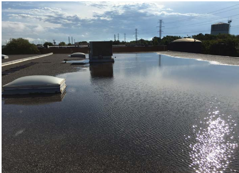
» This building suffered from leaks due to an improper draining system (above), until J Reynolds provided re-roofing and repair services (below).
