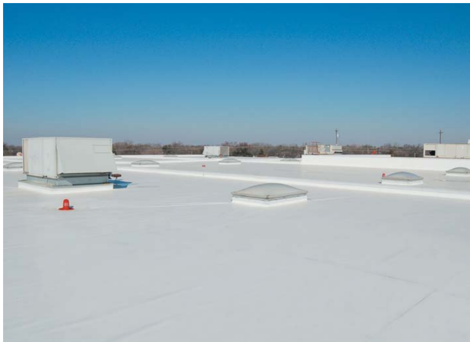
» This building suffered from leaks due to an improper draining system (above), until J Reynolds provided re-roofing and repair services (below).
