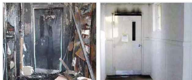
This properly working fire door contained the fire protecting people, equipment and the rest of the building.
