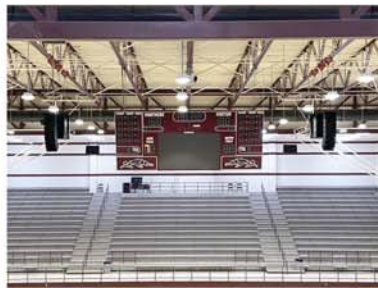
Dual RCF arrays, one for each side of the gym.
