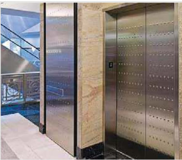
Elevator Shafts and Lobbies
