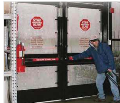
Delayed Egress Systems
