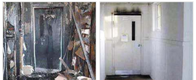
This properly working fire door contained the fire protecting people, equipment and the rest of the building.
