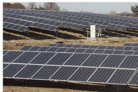
Johnson Controls also designed and constructed a 1,000 kW ground-mount PV system located at the Back River Waste Water Treatment Plant. Using SolarWorld modules and leveraging a grant from the Maryland Energy Administration, this project supports the City's objectives toward self-generation of 30% of all energy. This is a fixed-tilt, custom racking system suitable for the site's topography.
