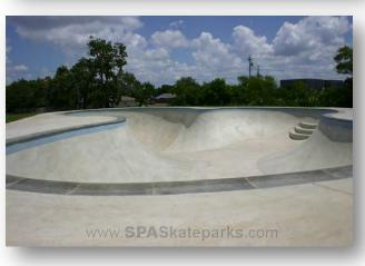
The transitional area of the College Station Skate Park consists of two unique bowls: a large, down-hill flow bowl and swimming pool replica. The flow bowl features a 10 ft deep end with a 14 ft extension, a bank wall, spine, and pool coping. The pool replica has an organic, free-flowing shape and features stairs, tile, and pool coping throughout.
