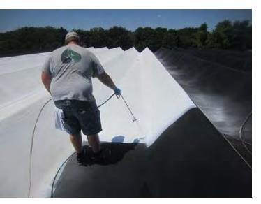
The final, and least expensive, option was to recover with the TRITOflex system directly over the Hypalon single-ply, avoiding thousands of fasteners with no seams and utilizing the existing membrane thickness to their advantage. In addition to that, a TRITOtherm top coat was recommended to repel ambient heat and also act as a sacrificial layer on top of the waterproofing membrane to create a roof that is sustainable for generations.
