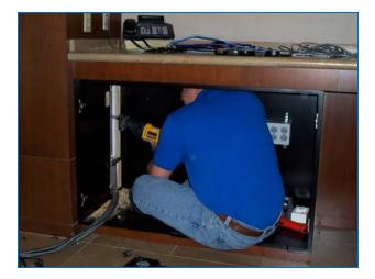
Installation begins with wall plates, speakers, and other "field" components. While a building project is in the rough phase, we install cables and mechanical equipment in preparation for the products to follow.
