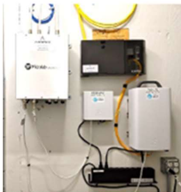
SAMPLE IDF WALL MOUNTED AIRWAVZ / CARRIER EQUIPMENT
