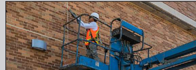
BUILDING & GARAGE RESTORATION
