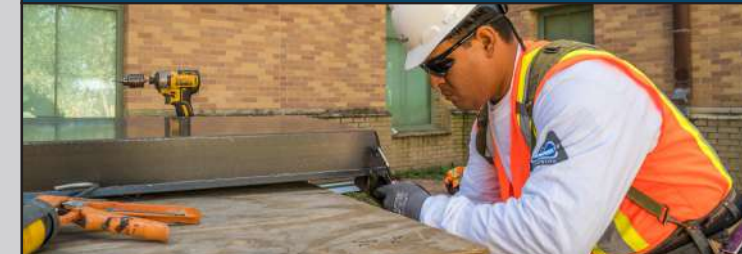
ROOF MAINTENANCE & LEAK REPAIR
