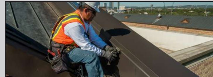
ROOFING & SHEET METAL
