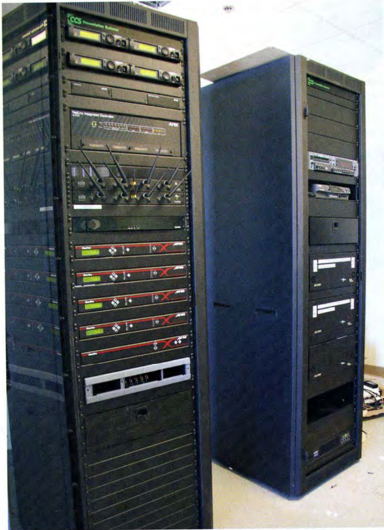
Two 44-space Middle Atlantic equipment racks house the bulk of the gear in SGA's Executive Boardroom—including Revolabs wireless receivers, an AMX NetLinx controller, Tandberg and ClearOne conferencing systems, an Altinex matrix switcher, a QSC CX204V power amp for the Tannoy sound-reinforcement loudspeakers, and ancillary equipment.
